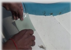
Align the sticky side of the Patch to the damage area
