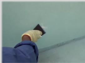
Firmly smooth the entire UV Patch to the damage area. Expose to daylight to fully harden
