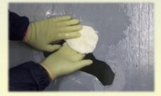
The final putty pouch is applied and compressed to close the hole
