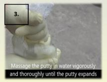
As the Putty expands form a putty ball shape. Then apply constant compression on the putty and the leak until the putty hardens.
