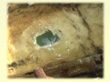
Hole Sealer Plug<sup>™</sup> requires constant compression over the leak until hard
