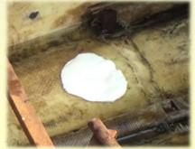
Hole Sealer Plug<sup>™</sup> fully cured. The putty contains Nano X5 which provides structural integrity
