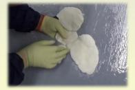
The putty is compressed both sides of the boat hull
