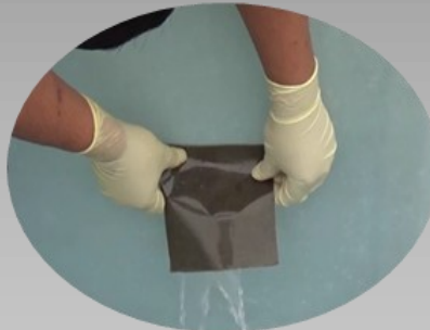
Apply PEM 'sticky' Patch Straight from the pouch
