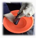
Quickly remove the Black Tape from the water and commence wrapping the Tape over the Putty
