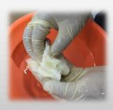
Wrap the Black Tape over the Putty starting from one end of the damage area
