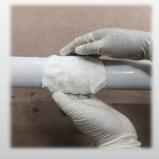
Repeat the spiral wrapping until a structural wrap is achieved. The putty should remain soft during the wrapping process
