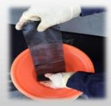
The Putty will migrate into and through the Black Tape providing a effective and strong repair after full curing and hardening
